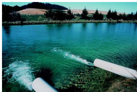
Excess water from the gold extraction process is treated and then held in this pool. It is checked to make sure it meets the required standard of purity before being discharged.
